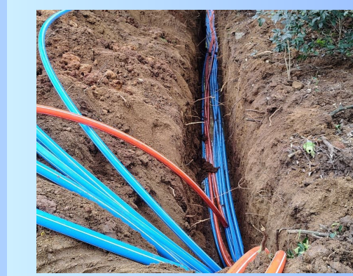
Underground MCF deployment
