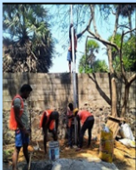
Aerial Pole installation
