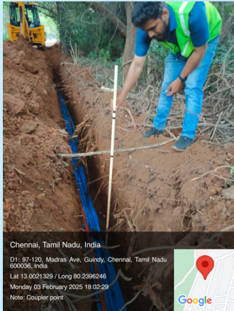
Trenching and ducting
